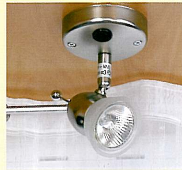
Directional halogen spotlights provide additional lighting. (1)
