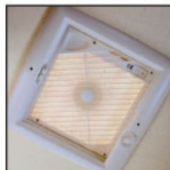
3 speed roof ventilator to all kitchen areas.
