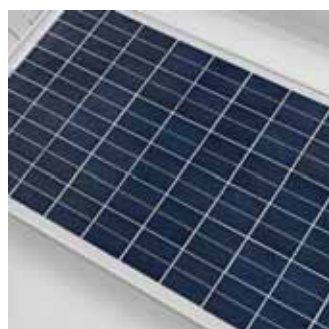
85 Watt solar panel installed
