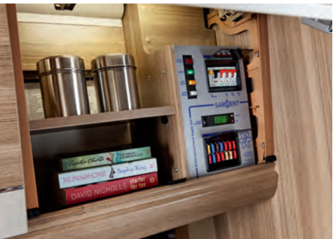
⚡ New: Eye level (not 749) consumer unit for the main 230V supply
