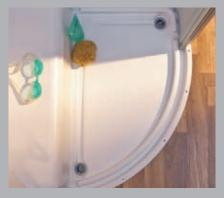
Optimal drainage guaranteed: All of the shower trays are equipped with two opposing drain holes. In this way, the shower water can also flow away quickly and without restriction if the vehicle is parked on uneven ground or on a gradient.
